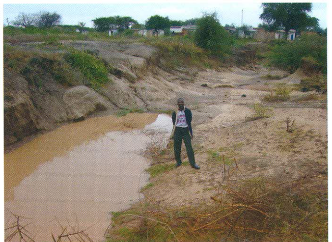
Erosion due to excessive rainfall in Kenya lowlands.
